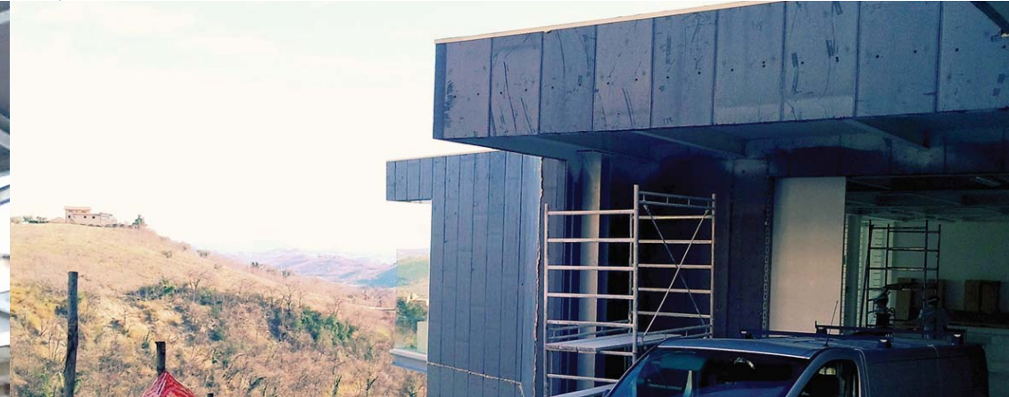
Partition panel laying
