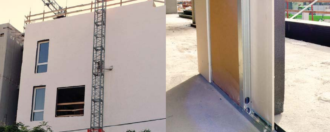
External insulation shaving finish
