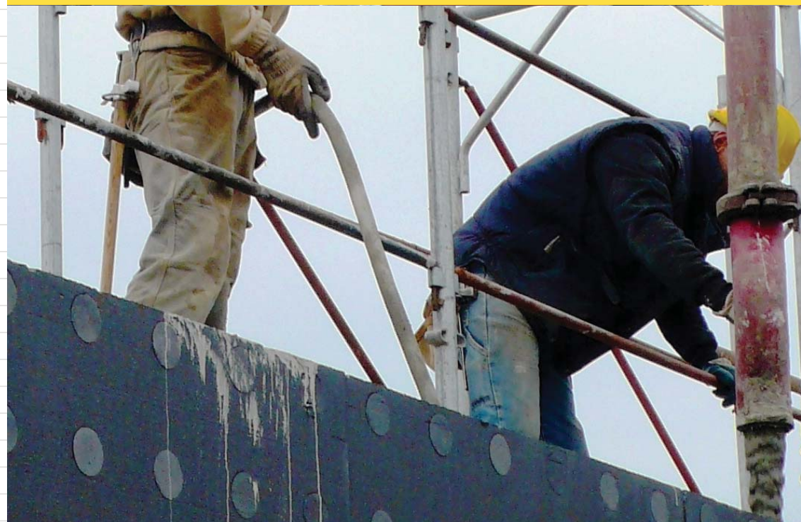
Beating on Wall Plastbau® 3 formworks by a wooden table and a rubber hammer while casting going up
