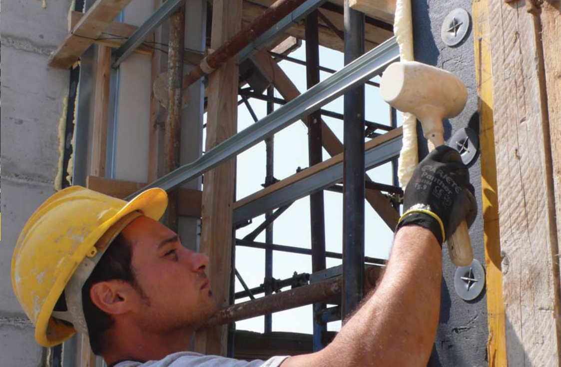
Beating on Wall Plastbau® 3 formworks by a wooden table and a rubber hammer while casting going up
