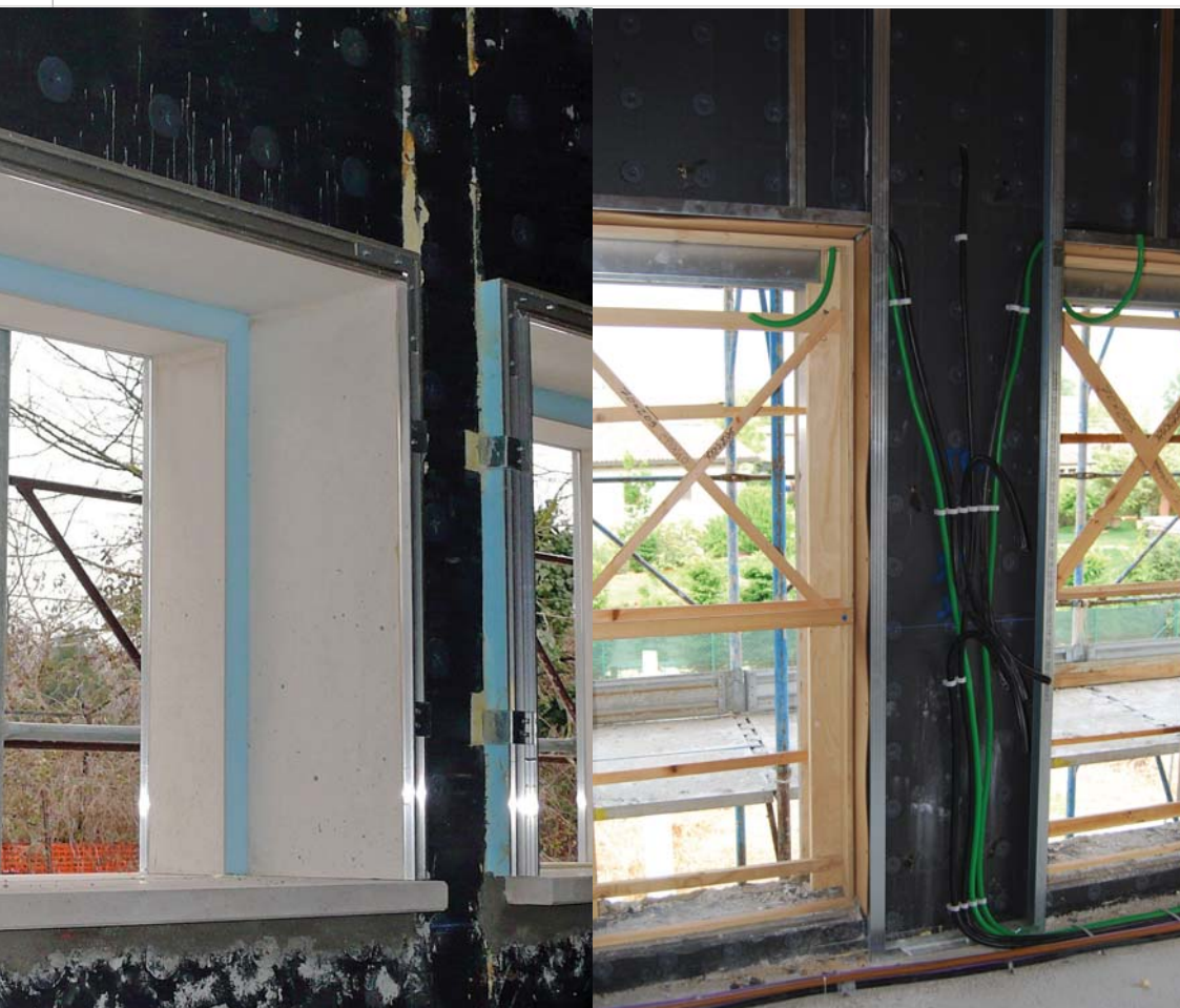
Prefab sub-frame to be mounted before casting
