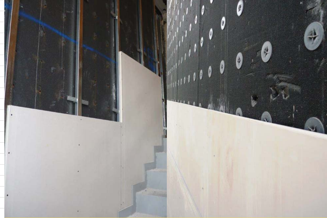
Plasterboard mounted on a structure
