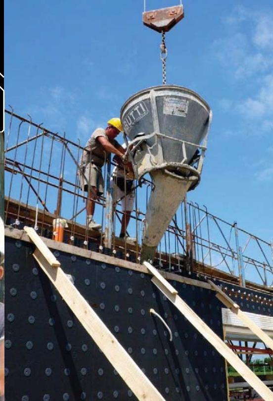
Casting with bucket
