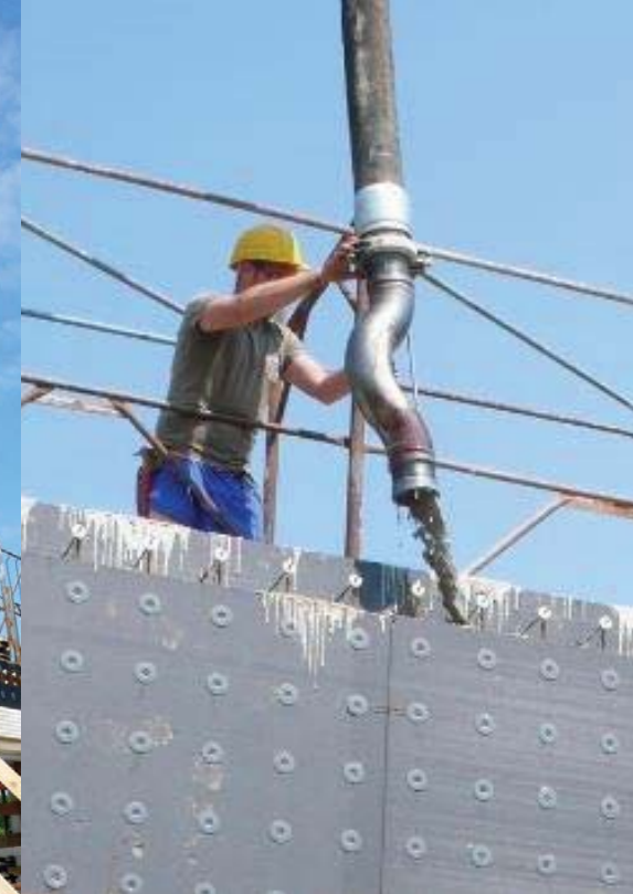
Casting with pump
