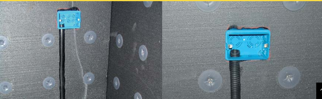
Installations, ducts on the Wall Plastbau® 3 internal panel
