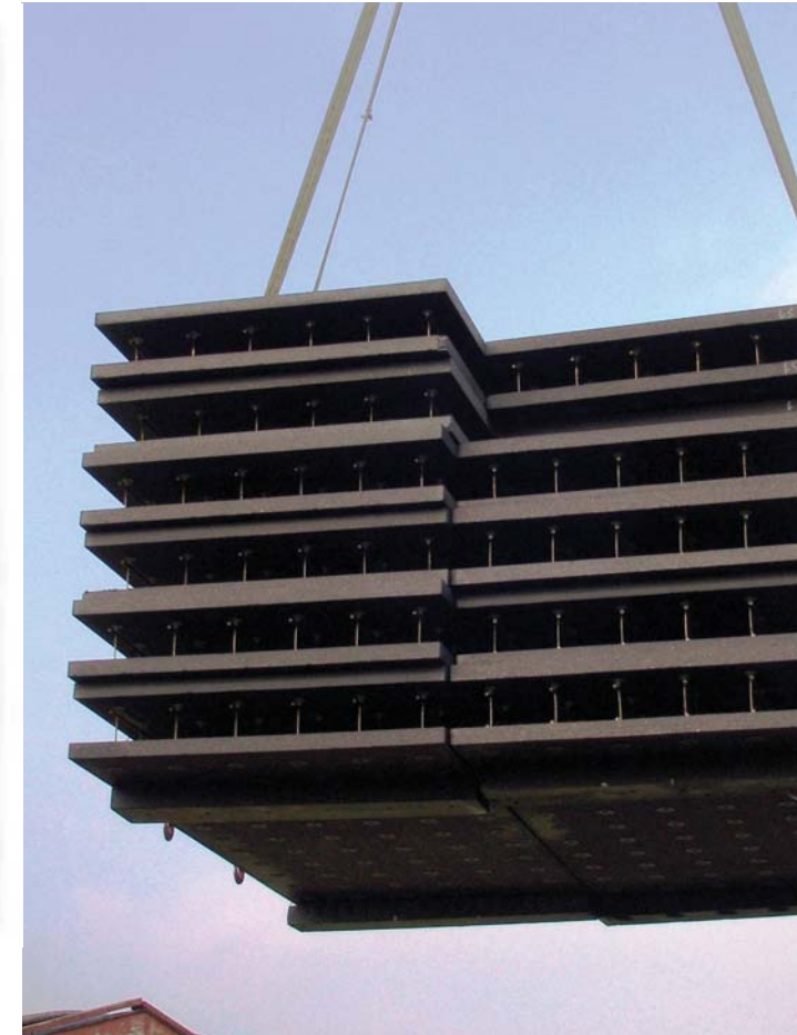
Unloading with crane
