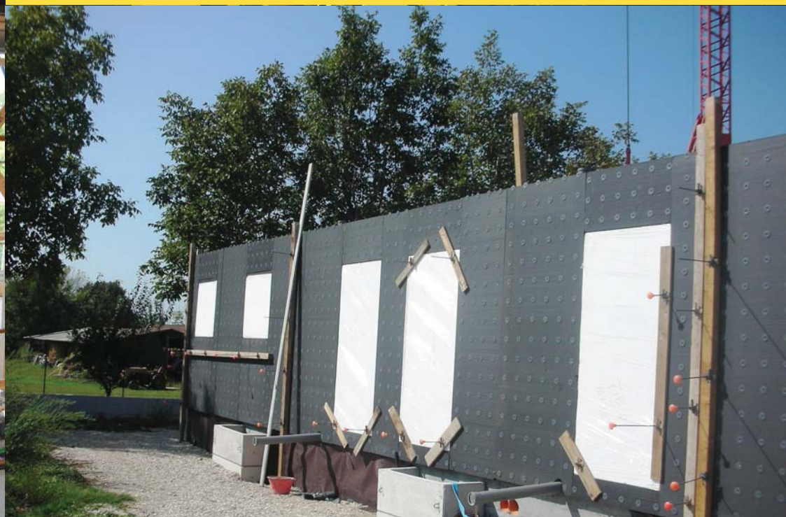
Mounting formwork with made-to-measure EPS blocks
