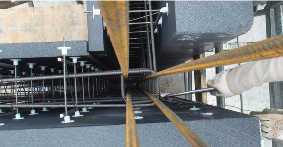
Semi-open corner node / reinforcement
